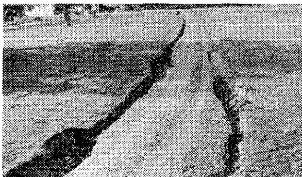
Erosion of farm tracks can severely limit access.
