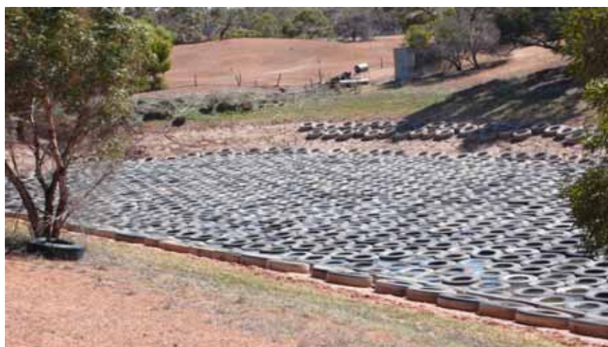
Tyres reducing dam evaporation on Buckleboo Station
